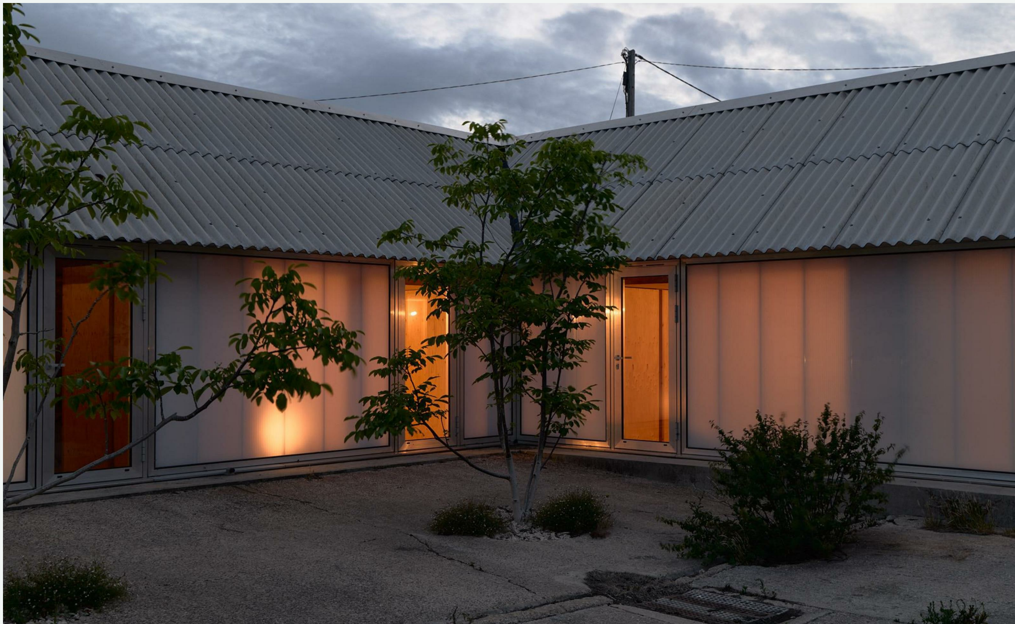
The Old Byre, Newport Road, Cowes, Isle of Wight
